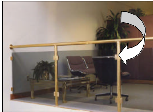
Metal Banister Bonded to Glass Panes with Tough, Durable DYMAX Multi-Cure ® 620
